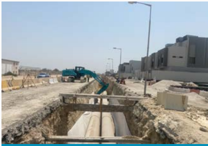
Stormwater Drainage Link
