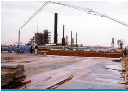
BAPCO NPCB Roof
