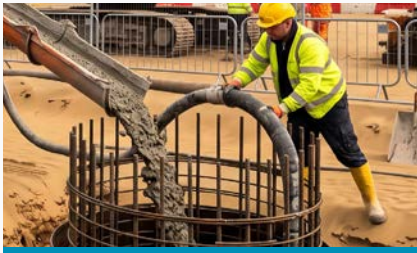
Piling Concrete
