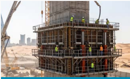
Slipform Concrete
