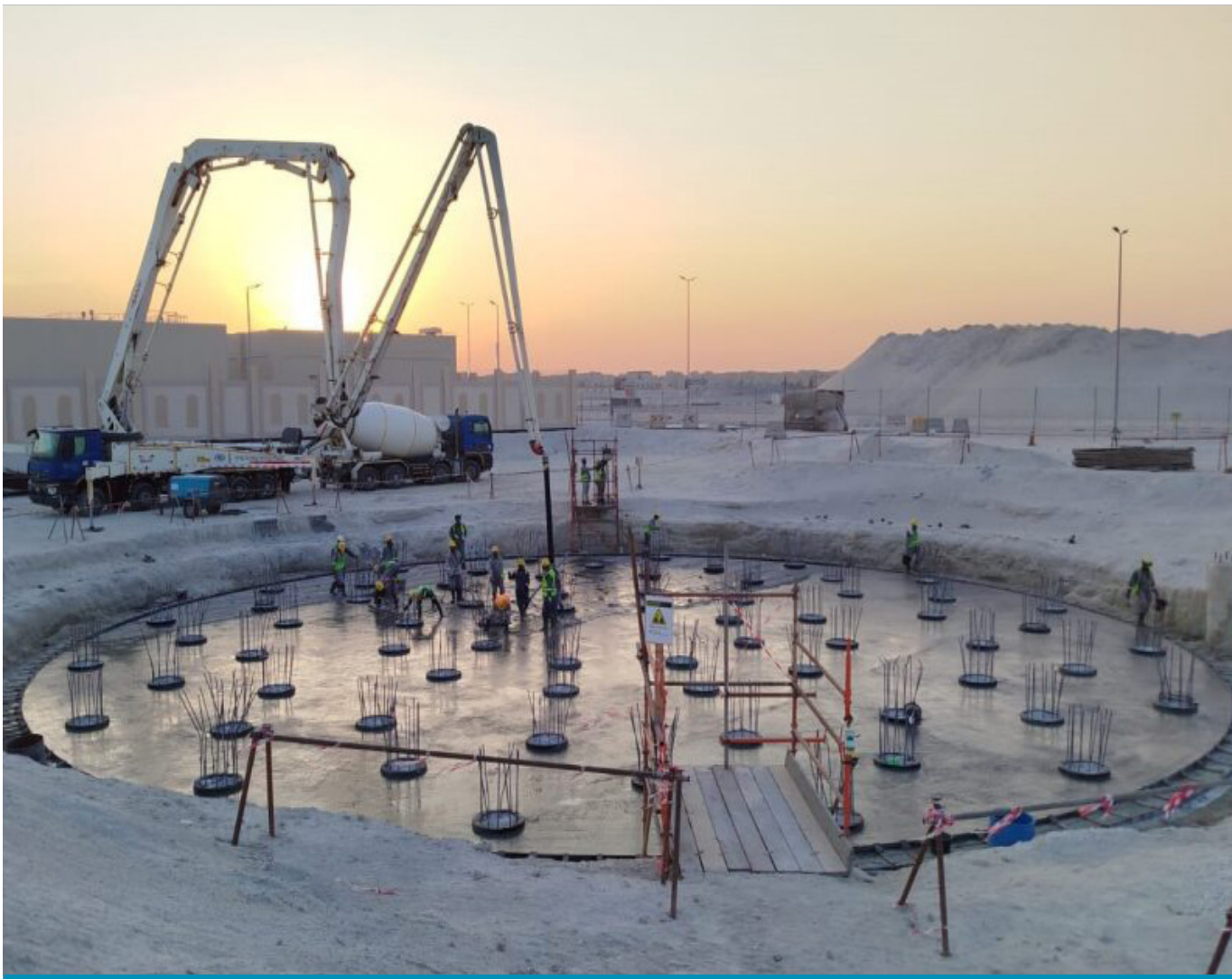
New Water Distribution Station East Riffa
