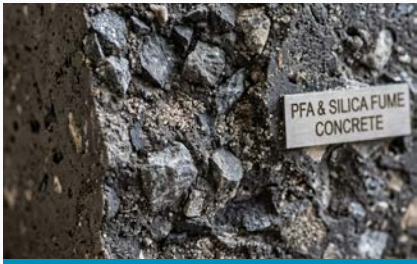
PFA & Silica Fume Concrete
